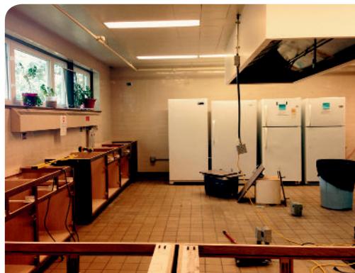
Kitchen renovation day 1
